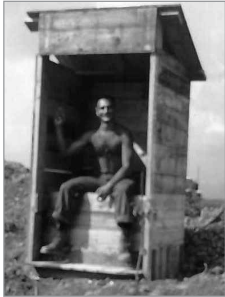
Latrine was made from ammo boxes. Originally no door but added later with hasp to protect.
