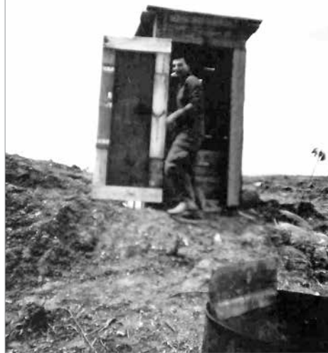
Latrine was made from ammo boxes. Originally no door but added later with hasp to protect.
